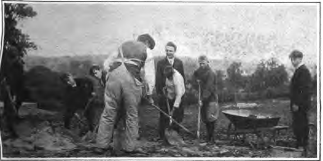
TEACHING THE BOYS TO MAKE CONCRETE IN SCHOOL DISTRICT NO. 8, TOWN OF GREENBURGH, WESTCHESTER COUNTY, N. Y.
